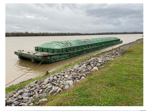
Photo 1 – Representative photo of the southern bank of the Arkansas River and current mooring at a deadman anchor (see steel cable on left side of photo) at Location 1. Replacement of 8 existing deteriorated deadman anchors with the installation of 22 mooring dolphins waterward of the shoreline will take place at this location.
